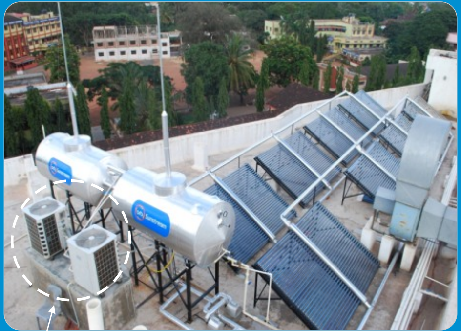
Sunstream 4000GM - Centralized System Integrated with Heat Pump
